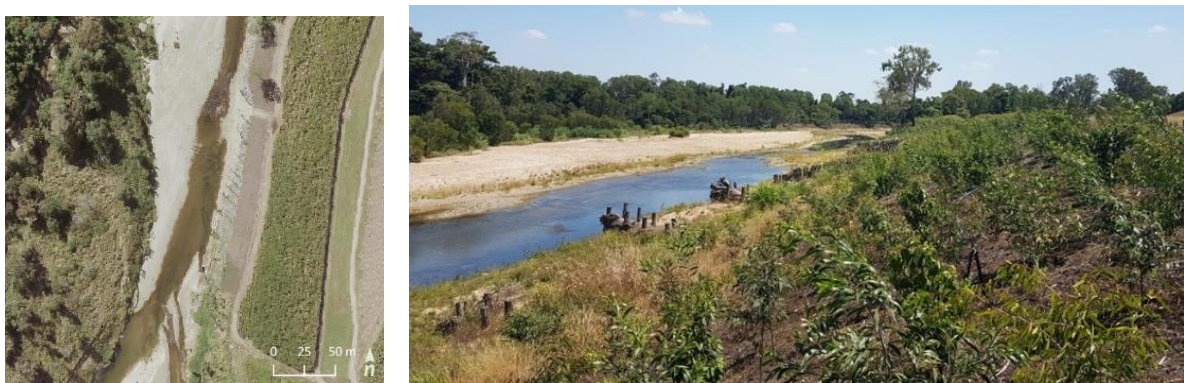
Figure 25. O'Connell River Site 2 pile field bank stabilisation. Aerial view (left), looking upstream (right).
