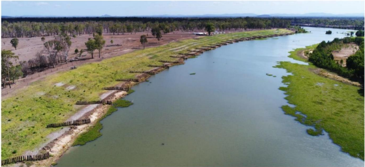
Figure 1. One of the largest river bank stabilisation project in Australia used pile field groynes on the Fitzroy River.
