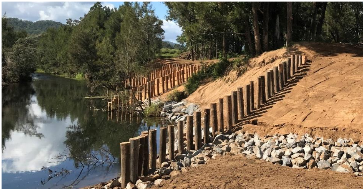
Figure 4. Recently constructed pile fields on the Mary River, Kenilworth.
