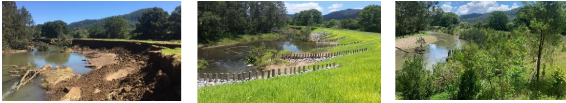
Figure 68. Vegetation establishment at a site over time following bank reprofiling and pile field installation, the photo on the left is 2017 and the photo on the right is less than five years later.
