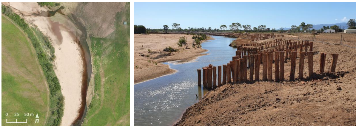
Figure 27. Molongle River pile field bank stabilisation. Aerial view (left), looking downstream (right).
