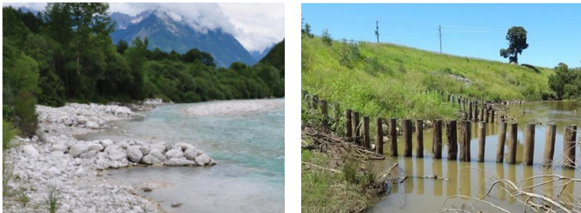
Figure 3. Example of impermeable rock groynes in Italy (left) (Sukhodolov, 2017), and permeable pile field groynes in Australia (right).
