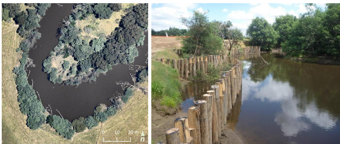
Figure 28. Yarra River pile field bank stabilisation. Aerial view (left), looking downstream (right).
