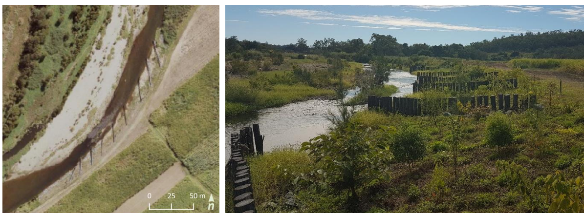
Figure 26. St Helens pile field bank stabilisation. Aerial view (left), Looking downstream (right).
