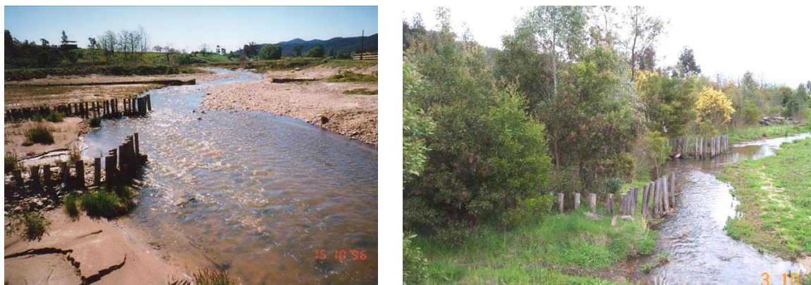
Figure 7. Example of vegetation establishment within the embayments of pile fields at Black Range Creek in North East Victoria.
