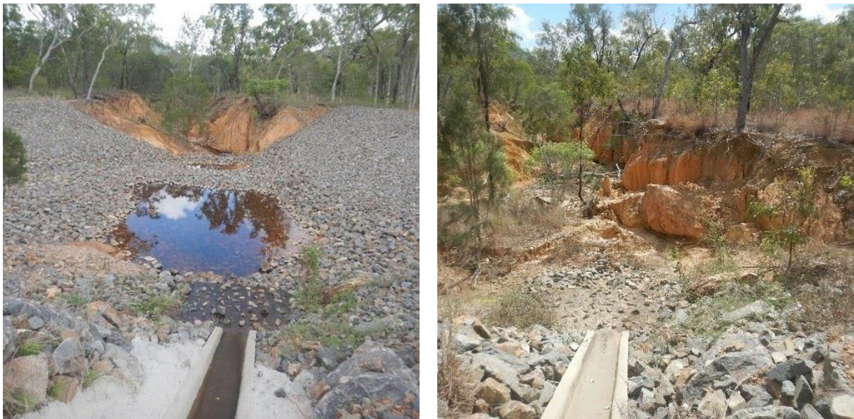
Figure 9. Before and after erosion control at site 8 road drain and gully, along Oaky Creek Road. (Photo credits: Jeff Shellberg)
