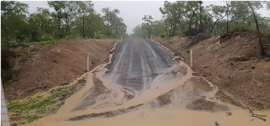
Figure 38: Table drains well connected to streams with few places to divert sediment laden water from bare batters.
