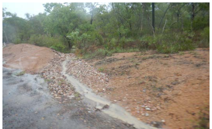
Figure 45: Small rock chutes at diversion drain outlets can prevent gully head-cutting upstream into drains.
