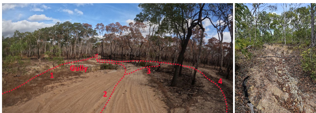
Figure 38 Track locations over 8 years avoiding a gully created by the track (above left). Abandoned track still eroding and unvegetated after many years (above right).
