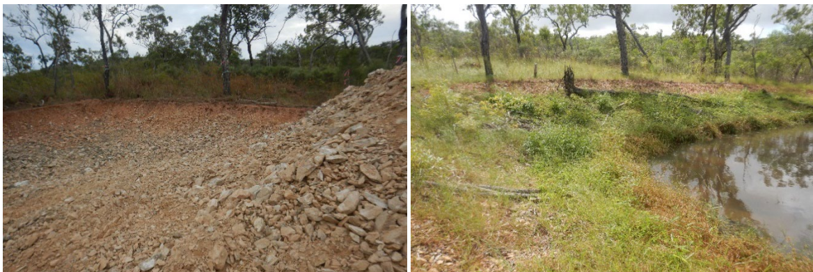
Figure 35 Source rock from local borrow pits on stable bedrock ridges (minimise area to 20 m x 20 m) and rehabilitate area after completion including any drainage erosion control.
