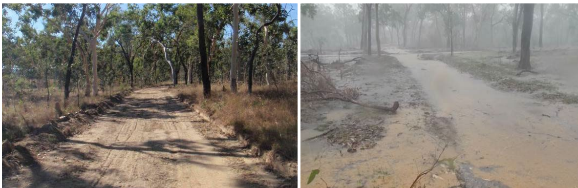
Figure 23 Grading the road down each year creates entrenchment and erosion.
