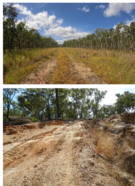
Figure 21 Primitive road locations on A) a stable ridge track with good grass cover and low maintenance (right above) and B) an unstable alluvial slope with chronic erosion along a fenceline track (right below).
