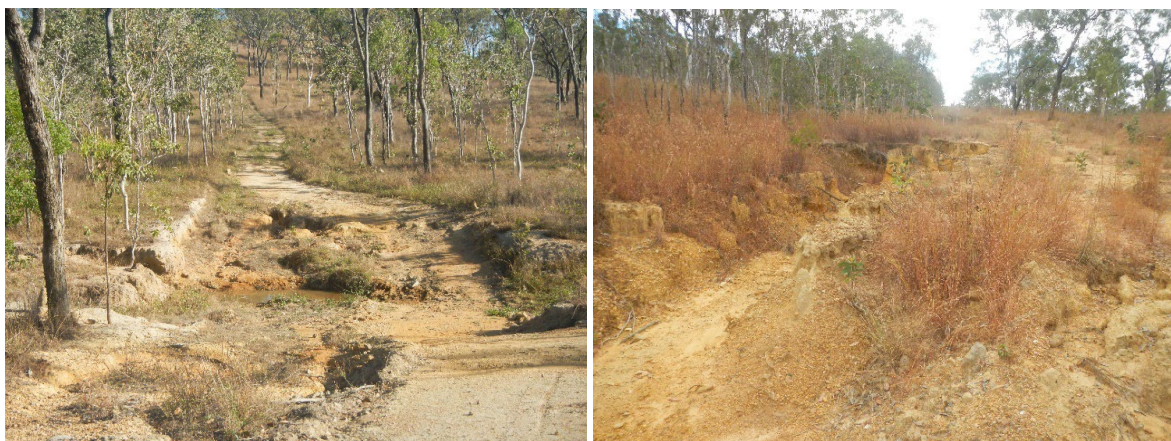
Figure 22 Typical eroded stream crossings and approaches along primitive tracks.
