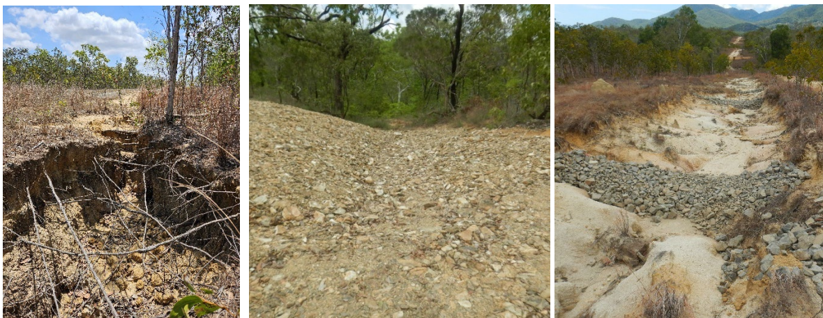
Figure 41 Road gully at a drain outlet (left) addressed with a rock chute (middle) to control flow energy. Check dams installed in an old track and gully (right).
