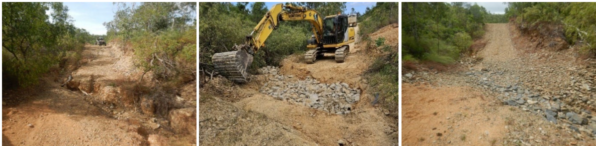
Figure 36 Before, During and After rock armouring of a gullied stream crossing.
