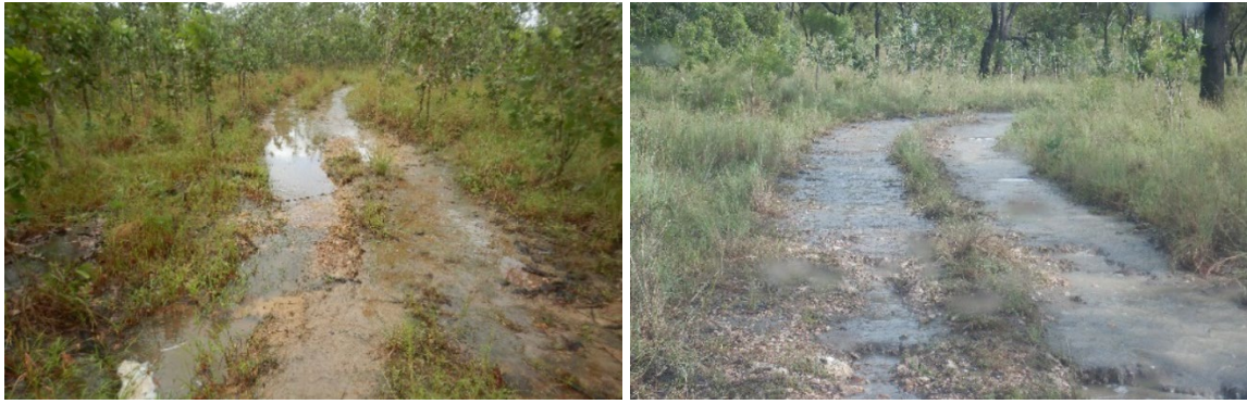
Figure 3 Typical primitive road (2-wheel dirt track) on CYP with intercepted water flow in the wet season.
