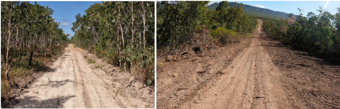
Figure 8 Typical annual grading along a fenceline that will accelerate wet season sheet and shallow rill erosion.
