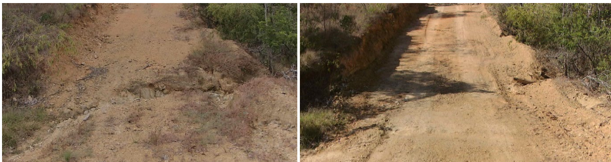
Figure 6 Annual grading before (left, June 2022) and after (right July 2022) track preparations for firebreak access. The cycle continues of erosion, re-grading for access, and re-erosion the next wet season.
