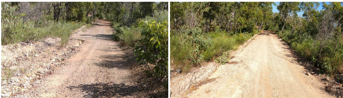
Figure 5 Annual grading before (left, June 2022) and after (right July 2022) track preparations for firebreak access, repeatably filling in erosion holes to be re-eroded the next year in the same location.
