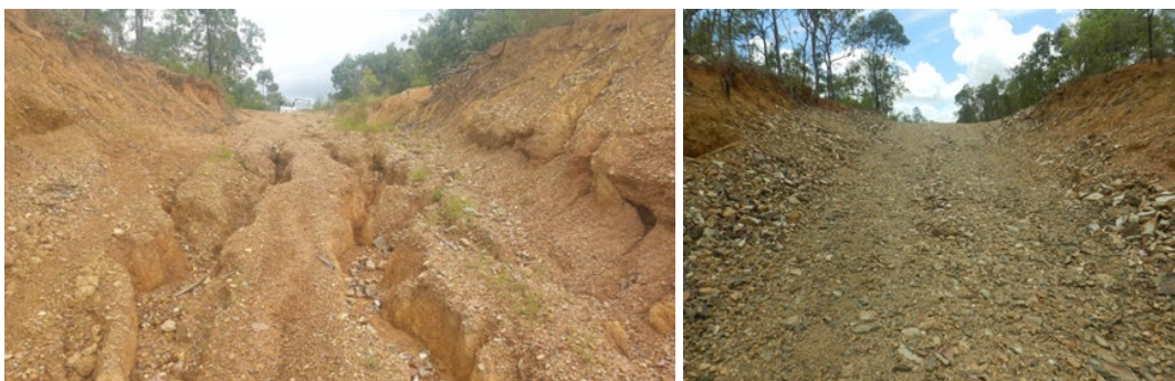
Figure 37 Before/After rock sheeting of a gullied road cut approaching a stream crossing.
