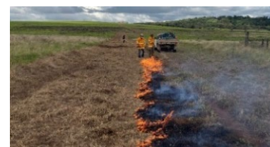
Figure 27 Two-wheel track firebreak with prescribed burning with water and blower support.
