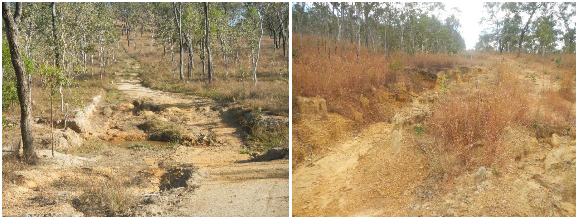
Figure 4 Typical primitive road gully erosion issues at small creek and hollow crossings.
