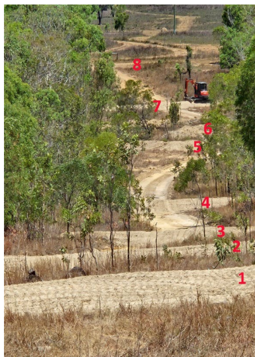
Figure 34 Example of water diversion banks (whoa-boys) sequentially installed every 30 m on a primitive track using local gravel/soil from ridgeline borrow pits.
