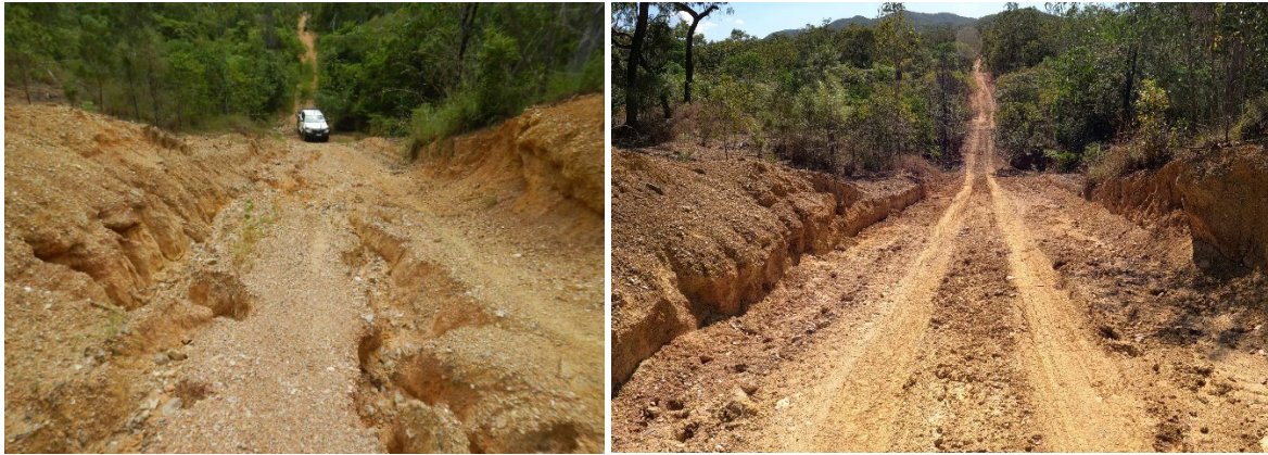
Figure 7 Annual grading before (left, June 2022) and after (right July 2022) track preparations for firebreak access. The cycle continues of erosion, re-grading for access, and re-erosion the next wet season.
