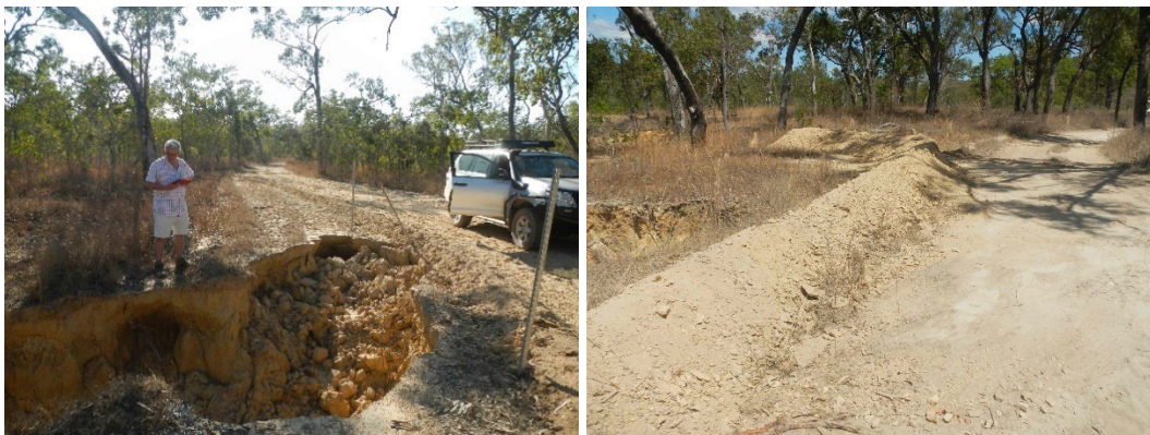
Figure 40 Divert water flow away from gully heads using water diversion banks (ridge gravel).
