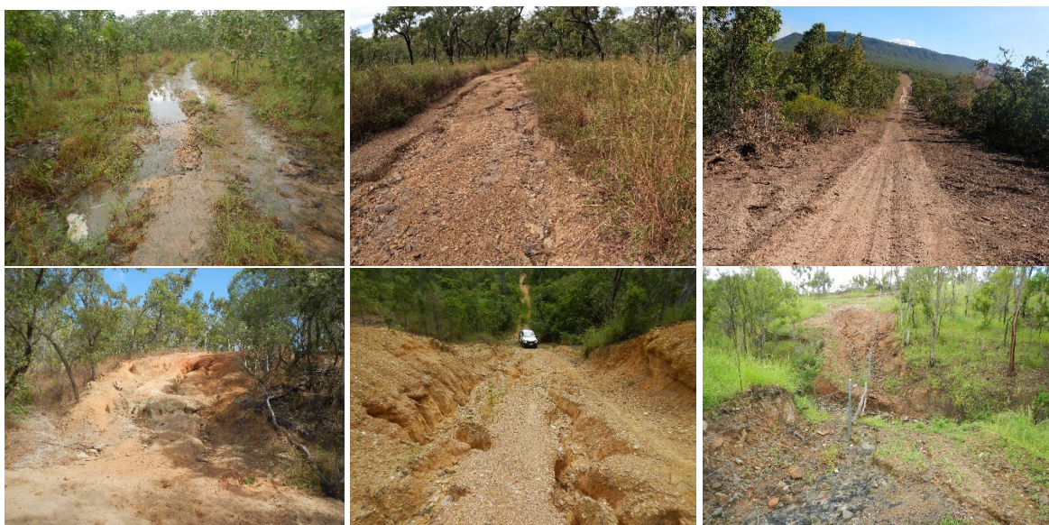
Figure 19 Examples of primitive track erosion issues across eastern CYP.
