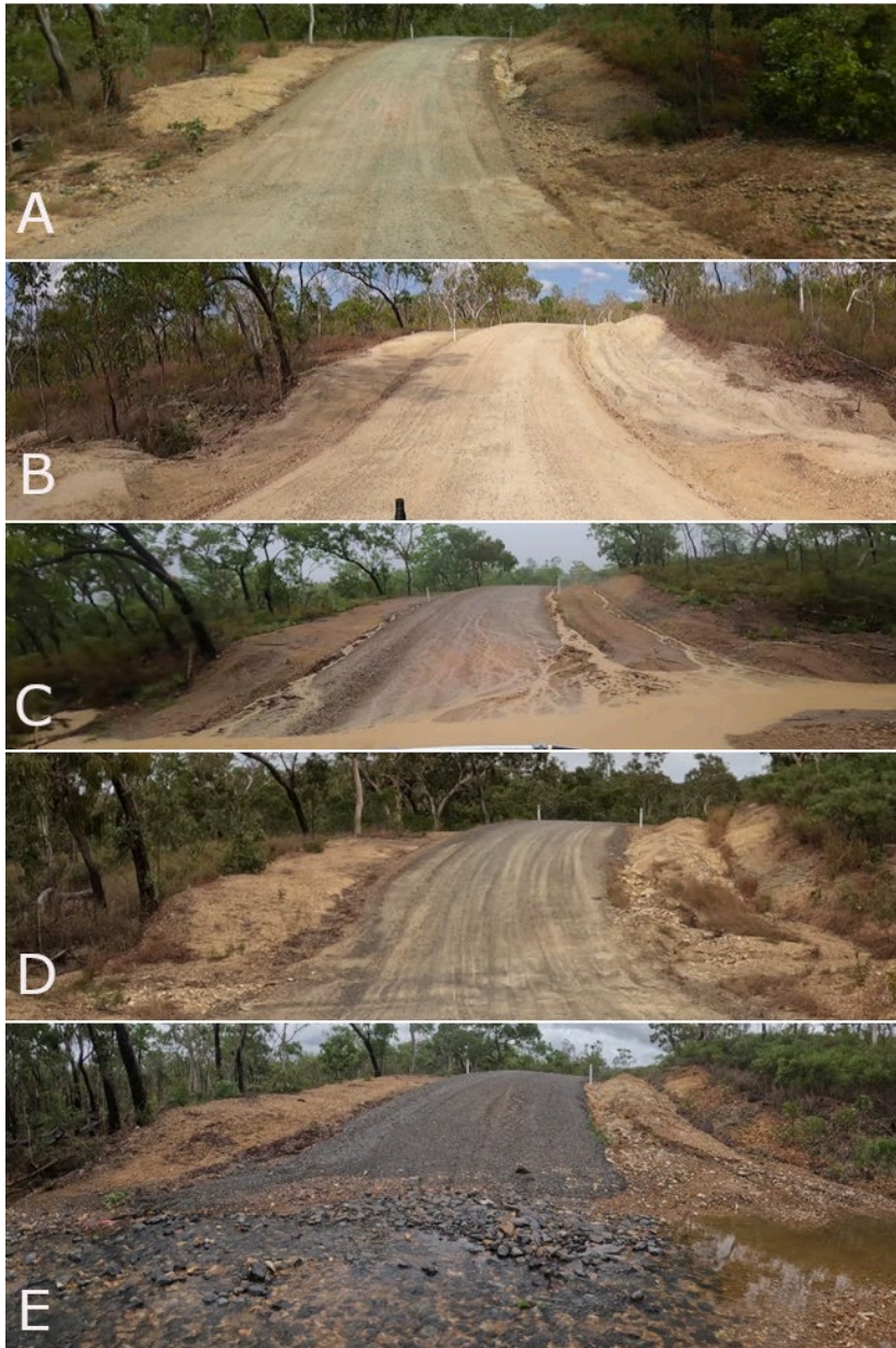
Figure 1 An unsealed road in July 2021 (A), Nov 2021 after DRFA works (B), Dec 2021 during a minor storm (C), June 2023 after an average wet season (D), and Dec 2023 after cyclone Jasper (E) showing the cyclic nature of maintenance and erosion
