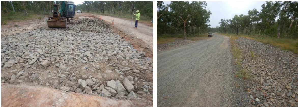
Figure 49 The coarse base of a rock crossing of a drainage swale and trafficable dip (left), inset into the existing road surface, with a thin layer of road base capping (right) that will settle into the rock below. The surveyor is standing on a bypass track which was later stabilised with rock mulch shown on the right.
