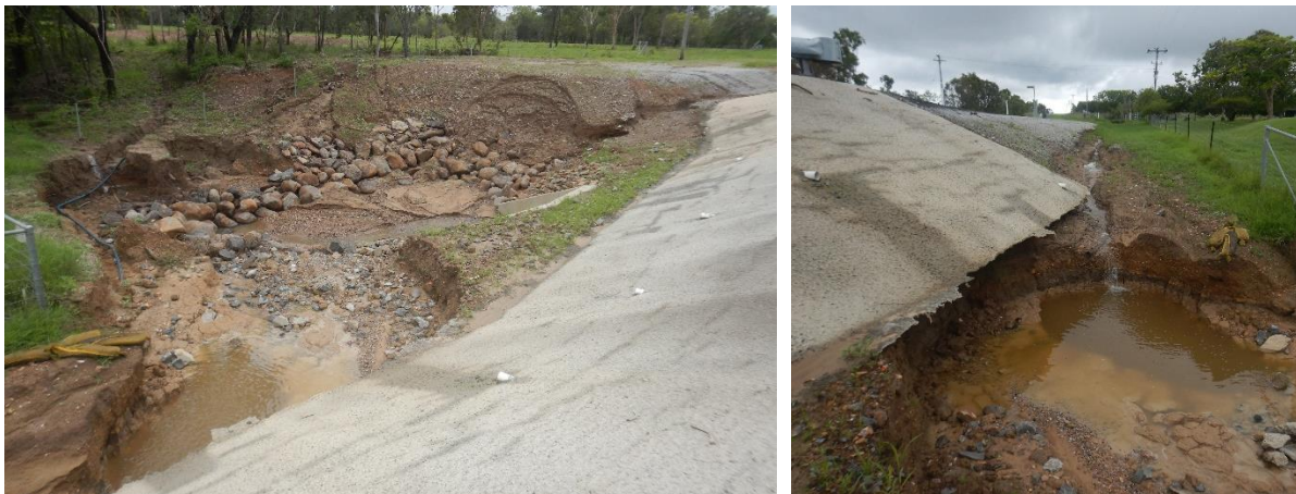
Figure 53 Inadequate rock erosion protection at the inlet of large box culvert, with associated gully erosion and slumping.
