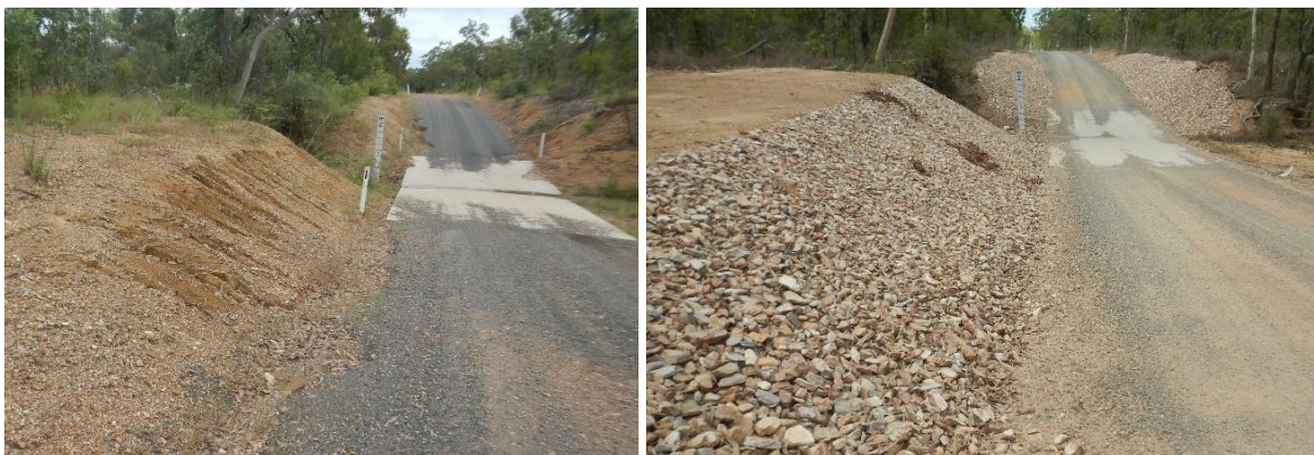
Figure 19 A batter with deep rilling in dispersive sodic soils (left) compared to the same slope with rock mulch (125 mm well-graded) applied (right).
