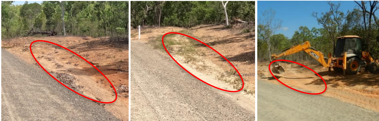
Figure 23 Hotspot of drain sedimentation (gravel, sand, and coarse silt > 20 \mu\text{m} ) before (left) and after (middle) the wet season, with subsequent silt removal with a backhoe along a 10 m drain length (right).
