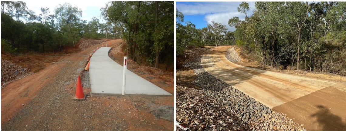
Figure 47 A concrete floodway poured in two (2) sections side by side to avoid the need for a temporary diversion track and associated erosion disturbance.
