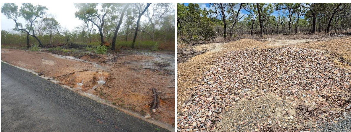
Figure 21 A clean water diversion drain re-entering the road batter and table drain causing gully erosion (left), and a small batter chute to control scour where clean water diversion re-enters the road system (right).
