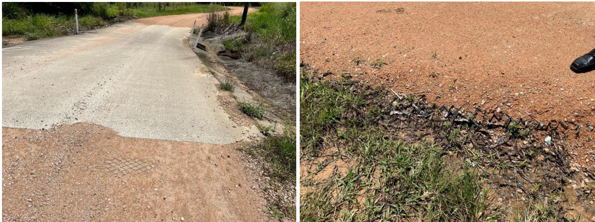
Figure 57 A cellular confinement systems (diamond shape) used to stabilise road base at an approach to a concrete floodway (Cassowary Coast Regional Council, photo Justin Fischer).
