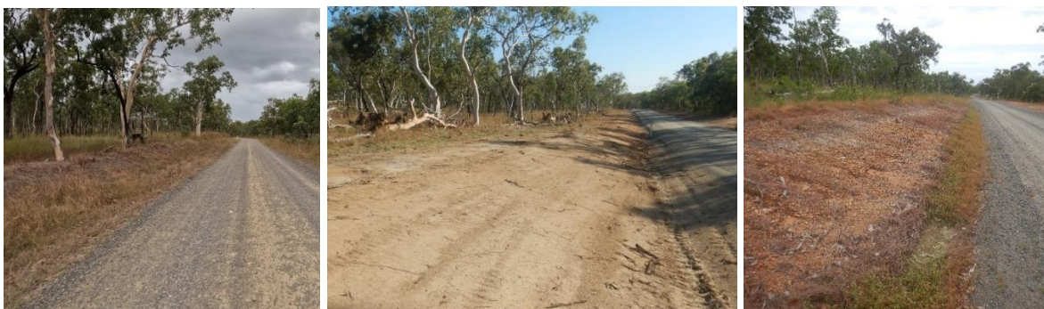
Figure 18 A stable grassed batter with native grass (left), that was re-sloped and graded with trees and grass removed down to sub-soil (middle), with subsequent rilling and sheet erosion from a longer slope length after one wet season and patchy grass colonization.
