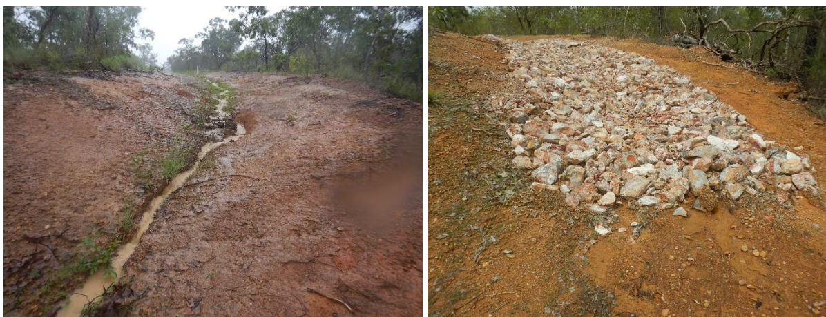
Figure 40 An incising V-drain outlet (left) and rock chute (right) at the same location to control erosion incision.
