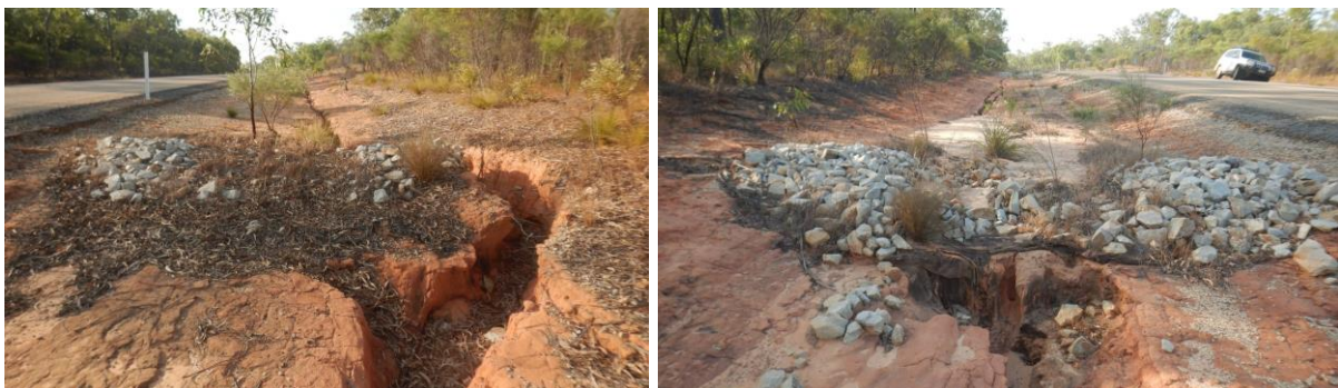
Figure 32 Failed check dams in non-dispersive soils due to outflanking (left) or excessive plunge pool scour (right) due to insufficient width up the drain batter (left) or insufficient frequency of check dams (right), note absence of check dams in the upstream direction.
