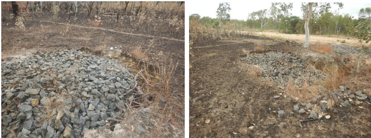
Figure 42 Failed rock stabilisation due to use of porous coarse rock (screened rock) in gully heads in dispersive soils. The gully head will seep and migrate around the rock unless a proper rock chute is shaped, layered and constructed (Figure 44).
