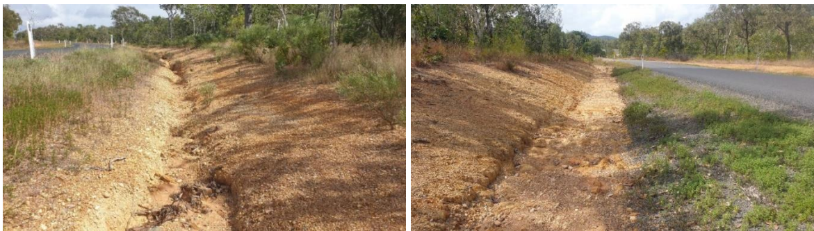
Figure 25 A V-Shaped Table Drain with erosion (left) versus a Flat-Bottom Table Drain (Trapezoid-Shaped) (right).
