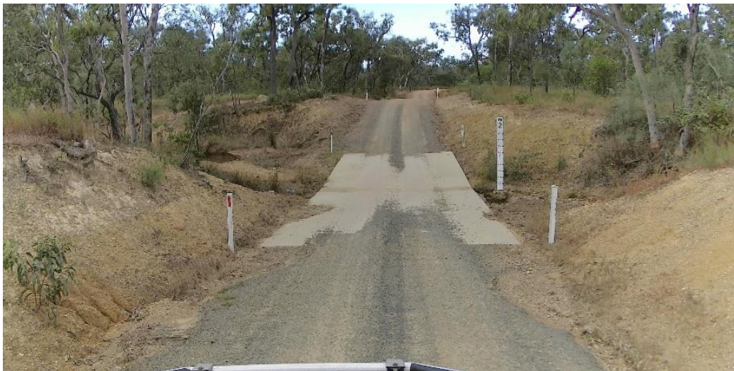
Figure 46 A concrete floodway installed at a creek crossing to reduce bed scour, but with associated erosion at the diversion track (Figure 50). Note downstream scour below concrete due to lack of rock protection; and rill erosion on batters.
