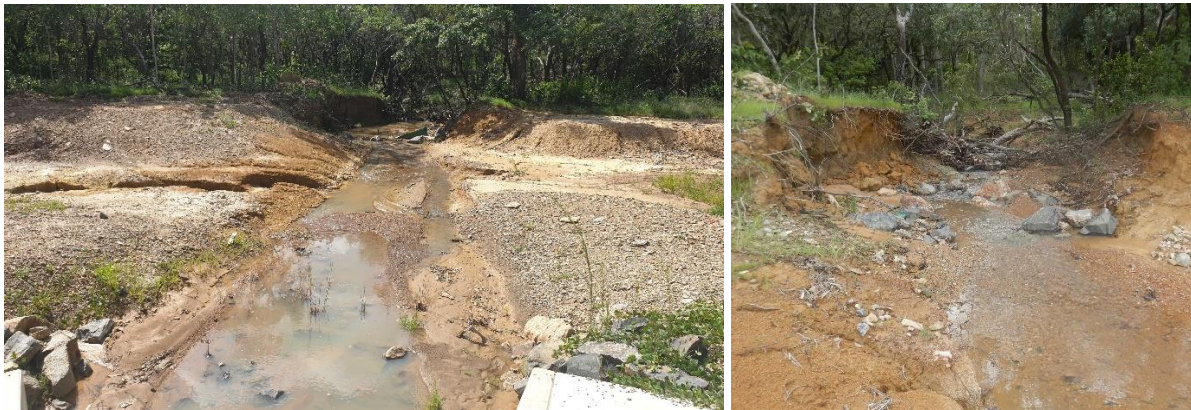
Figure 52 Minimal erosion control measures downstream of a concrete culvert, including a lack of rock protection and collapsed grade control structure and silt fence that were inadequate for the catchment area.
