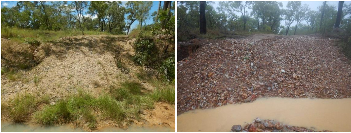
Figure 50 Deep rilling of a temporary bypass road crossing a creek (left) used during construction of a concrete floodway. Rock mulch placed on the same bank to mitigate soil erosion (right).
