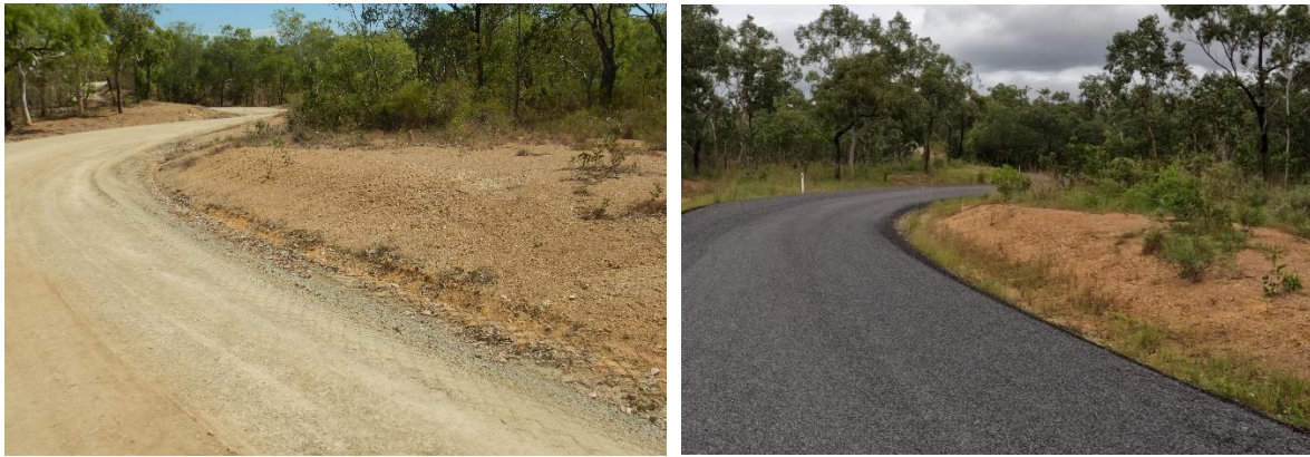
Figure 55 An unsealed road and stream crossing approach before (left, 2023) and after (right, 2024) a two-coat seal on top of a heavy formation grade (batters and drains left ungraded).
