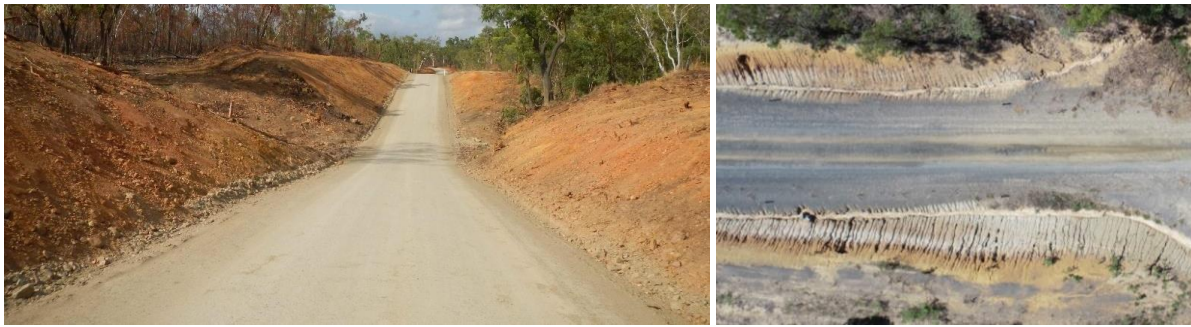
Figure 17 Some steep slopes are difficult to lay back without major bulk earthworks, and need to be stabilised in place with native vegetation, rock mulch, and/or chemical treatments.
