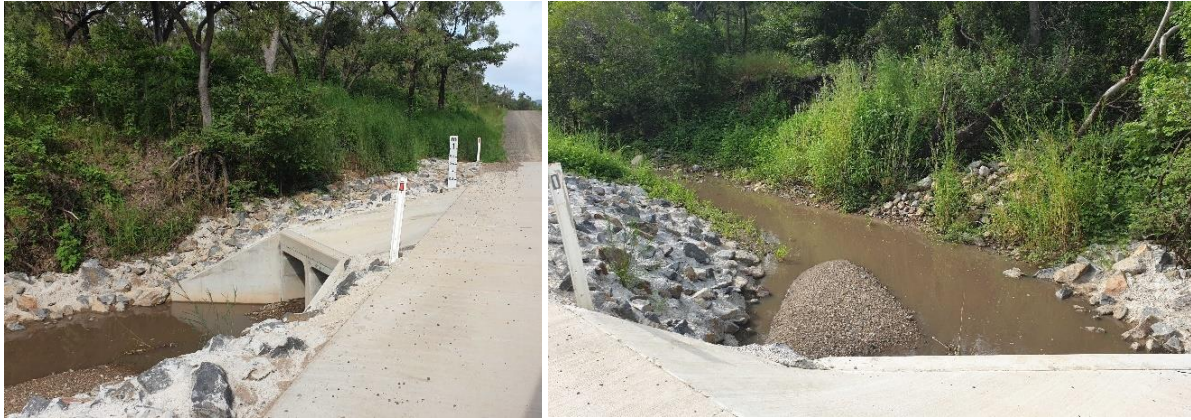
Figure 51 A well armoured box culvert with rock/concrete mix (left), but a lack of rock scour protection on the outside creek bank downstream (right).
