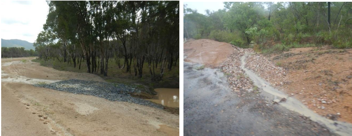
Figure 41 Small rock chutes at diversion drain outlets can prevent gully head-cutting upstream into drains.
