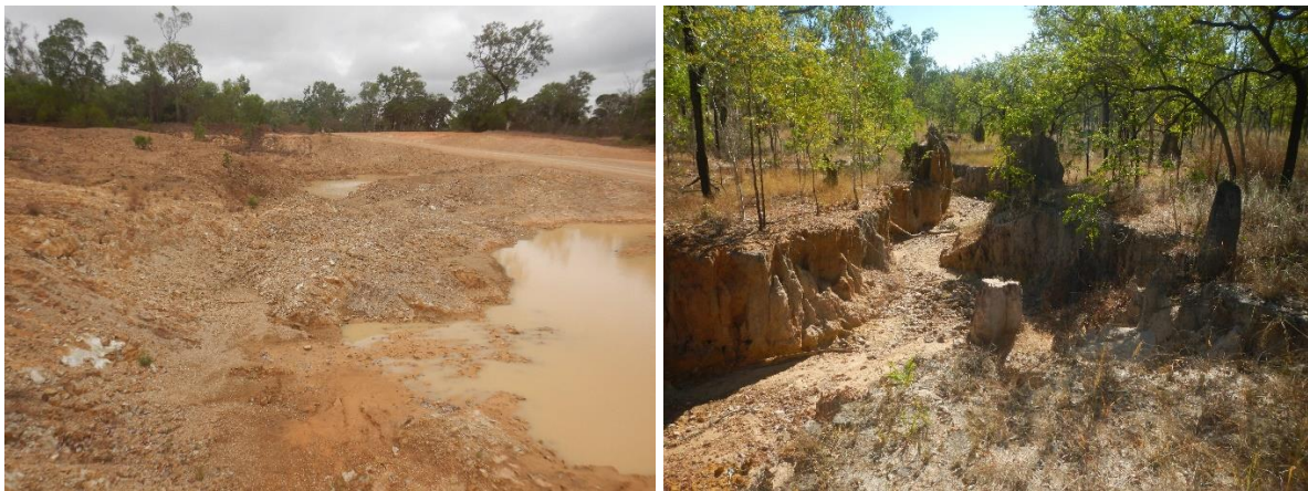
Figure 60 Abandoned gravel pit without proper rehabilitation and turbid rainfall runoff (left) and outflows causing downstream gully erosion and sediment pollution (right).
