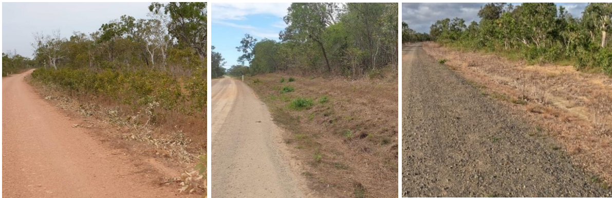
Figure 12 A stable roadside batter with tree sucker regrowth and good grass cover (left) that needed either slashing with a tractor (middle) or broadleaf herbicide application to avoid soil disturbance from grading.
