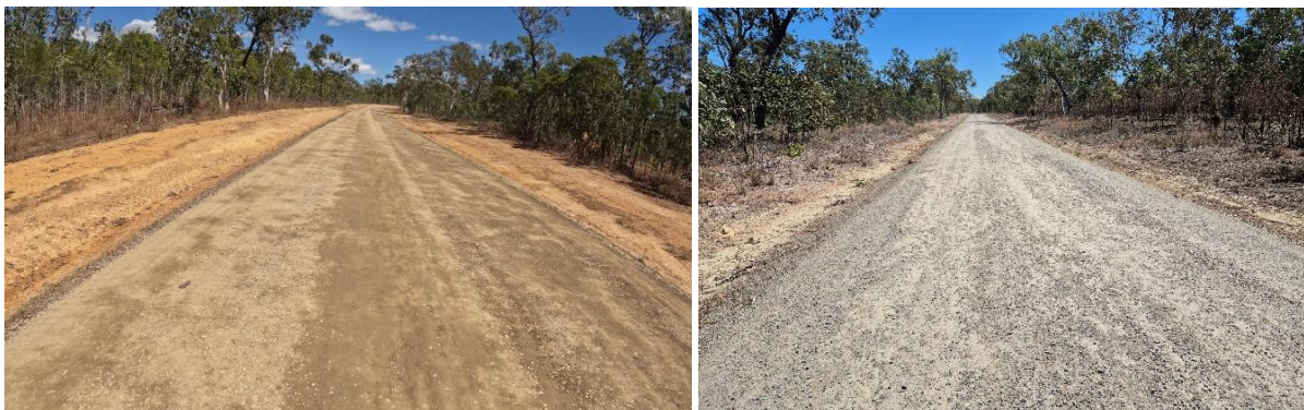
Figure 11 Unsealed road just after full maintenance including batter disturbance (left) and the same section a year later just after maintenance with no grading disturbance on the batters and drains.
