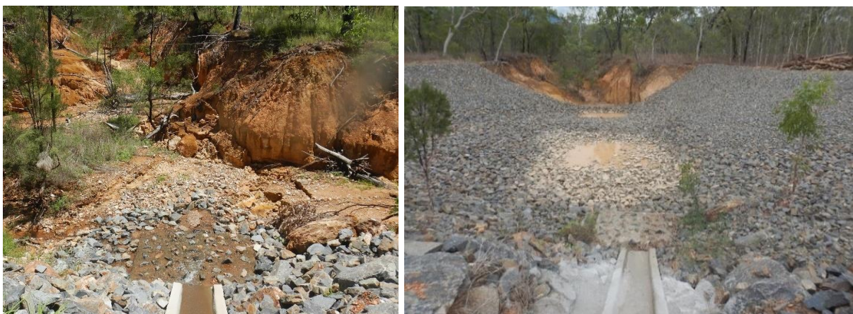
Figure 45 Gully bank collapse downstream of a concrete culvert and concrete chute due to a lack of rock scour protection in the receiving environment beyond the immediate structure (left), and after gully control and rock chute installation (right).
