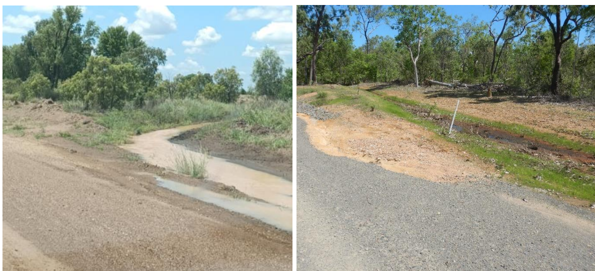
Figure 33 Diversion drain with an earth bund to turn runoff away from the road (left) and a breached earth bund due to drain sedimentation from a large drain catchment and inadequate drain slope and flow capacity (right).
