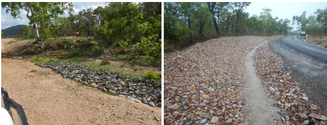
Figure 28 Rock-lined table drains on unsealed roads.
