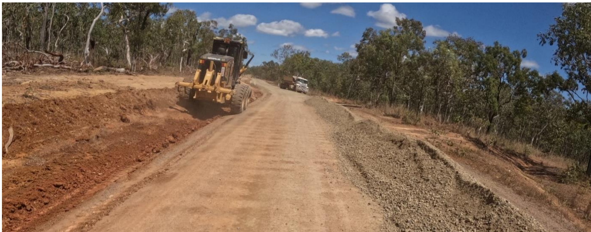
Figure 7 Typical maintenance work and medium formation grading on an unsealed road.
