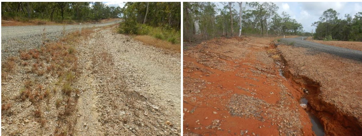
Figure 22 A functional semi-stable drain that does not need grading maintenance (left) compared to an unstable drain needed erosion control (rock) maintenance rather than just re-grading (right).
