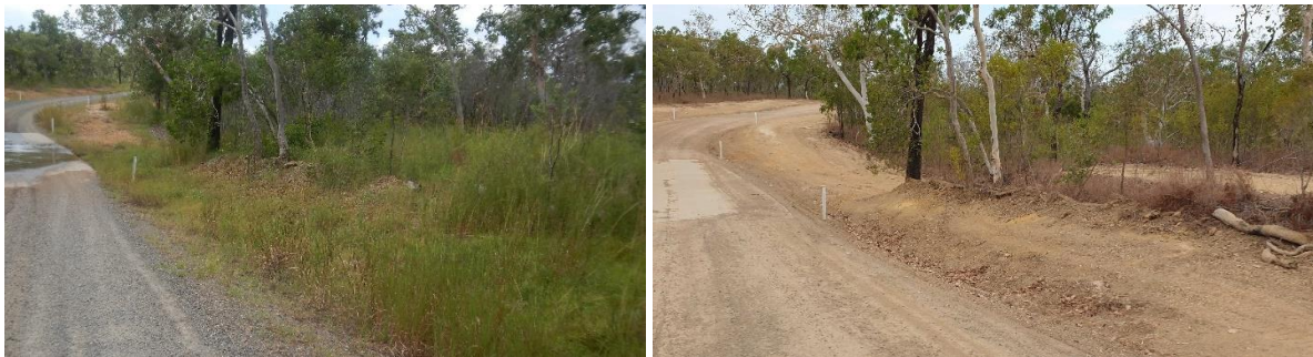
Figure 16 Batters with native grass cover retained for erosion control over multiple years (left) will be more stable than if annually graded (right).
