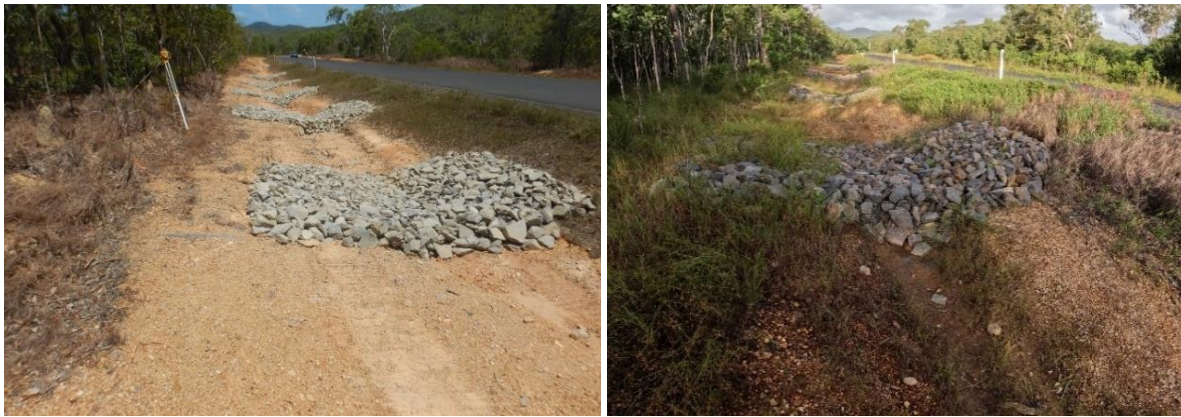
Figure 30 Check dams at the correct frequency and 0.5 % grade line between the crest of the downstream check dam and toe of the upstream check dam. Before (left) and after (right) a major cyclone. Note dumpy level on left used in construction.
