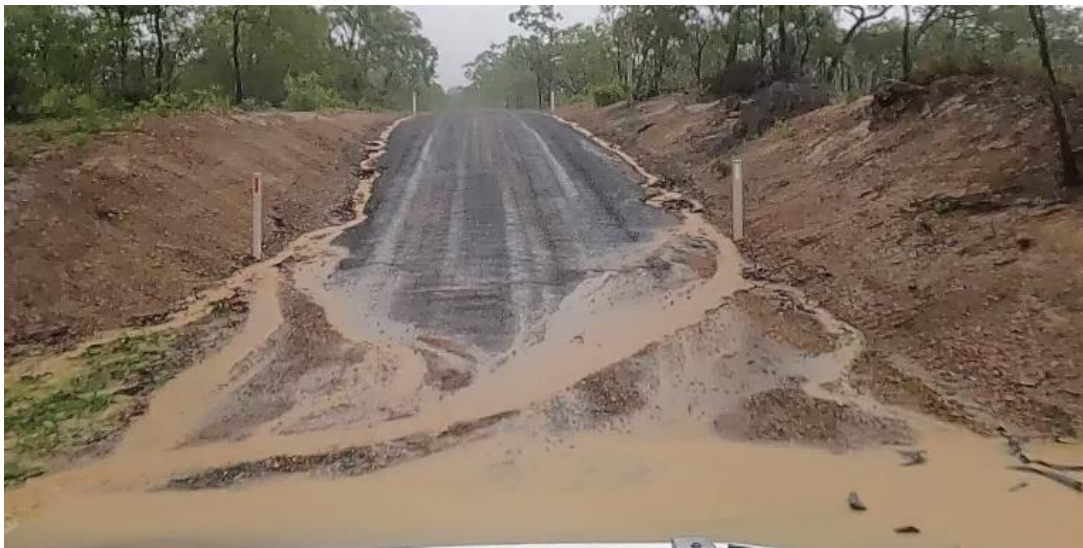
Figure 35 Table drains well connected to streams with few places to divert sediment laden water from bare batters.
