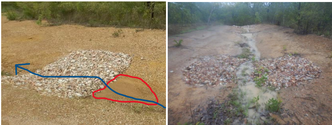
Figure 31 Sequential low-profile rock check dams in V-drains can control the slope and channel erosion without blocking drains or backwatering the road.
