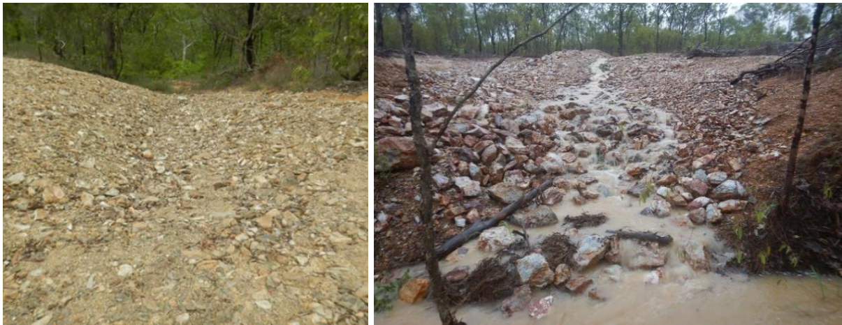
Figure 43 Rock chutes constructed at the outlets of road diversion drains to control gully erosion.
