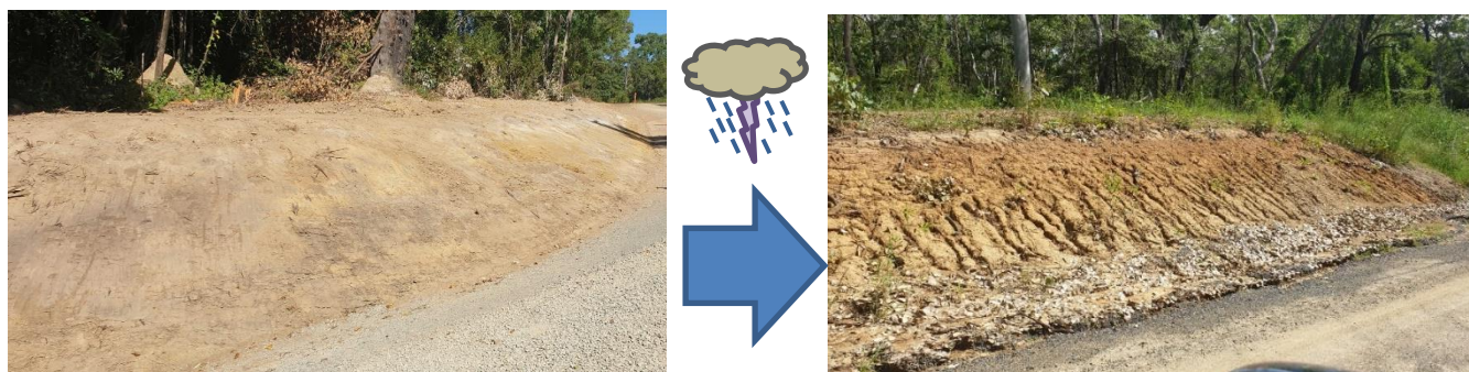
Figure 9 Dispersive sub-soils (score 3) at a road cutting with rill erosion one wet season after grading, with no vegetation growth or colonisation due to the harsh soil environment and erosion.
