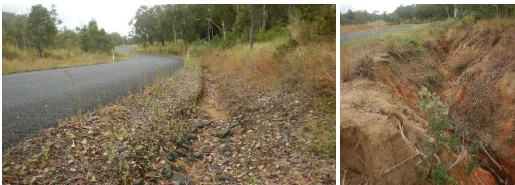
Figure 56 A bitumen 'dust seal' for community amenity on an existing alignment with sodic soils. Note untreated gully on drain outlet threatens road stability and reef health.
