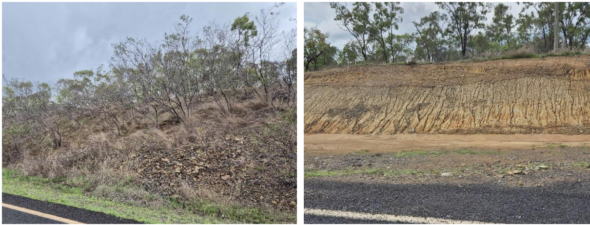
Figure 20 Rock mulch over sodic dispersive soils after 10 year of vegetation colonisation (left), and the same untreated soils (right).
